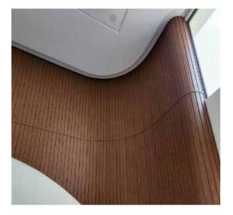
The Infratop system can be used on unusual surfaces. The panels and finishes are flexible, which allows, for example, to finish arches and curved walls.
